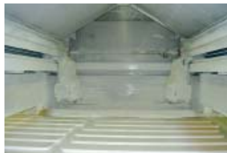
Two large sprayer heads paint the wood products as they pass through the spray line.
